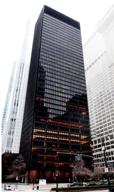
Source: Looking Back at One of Mies van Der Rohe's Most Famous Buildings (hyperallergic.com)
