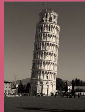
D. Leaning tower of Pisa, Italy
